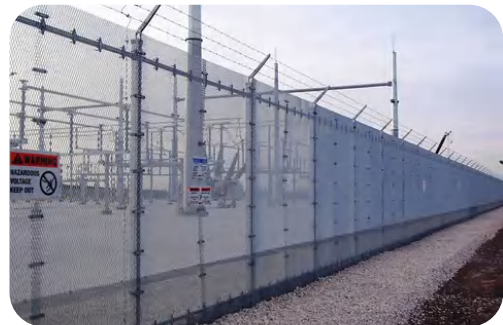
Expanded metal fence with barbed wires in the substation
