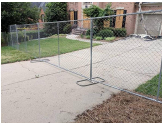
Demolition Sites Temporary Isolation
